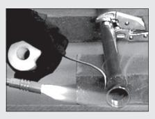
Solder a short length of pipe (about a foot or so) to a threaded adapter using only 95/5 tin-antimony or equivalent solder. Attach the threaded adapters to the water heater's connections (using thread sealant tape or pipe joint compound). Connect the home's water pipes by soldering, keeping the connections at the water heater cool with wet rags.
