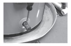
Figure 20 - Draining the old water heater.
