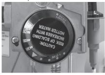
Figure 32 - Gas control/valve in Pilot Lighting position.
