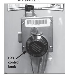
Figure 17 - Turn gas control/temperature knob OFF.
