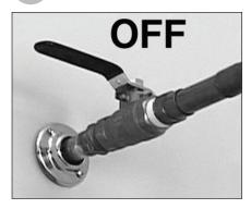
Figure 19 - Cold water supply in off position.
