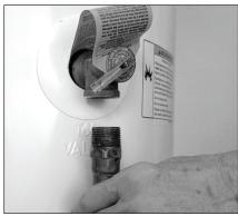
Figure 21 - Removing the T&P Relief Valve discharge pipe.
